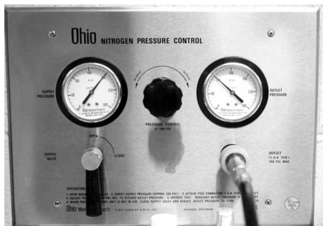
Figure 89-2 OR wall outlet for nitrogen gas.
